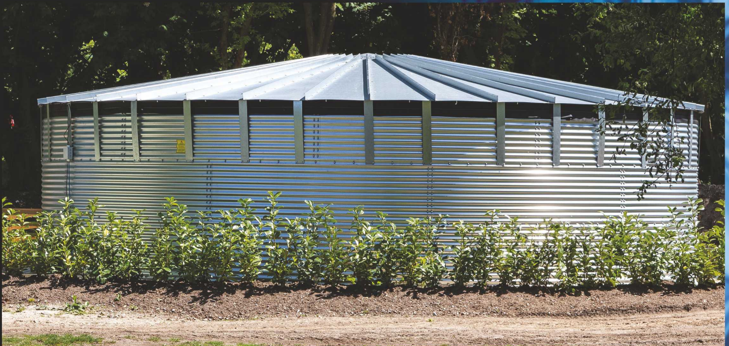
Typical Liquidrum® tank installation with 30° pitch steel cover
